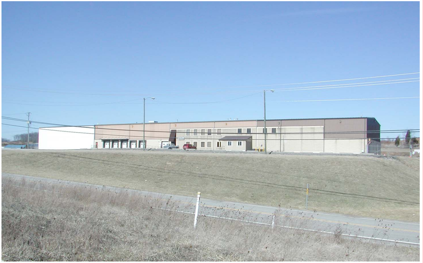
FRONT VIEW OF BUILDING
